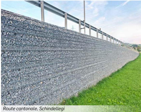
Route cantonale, Schindellegi
